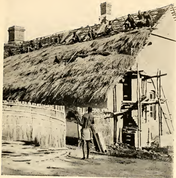
RE-THATCHING AN OFFICIAL'S HOUSE. C. Gouldsbury, phot.
